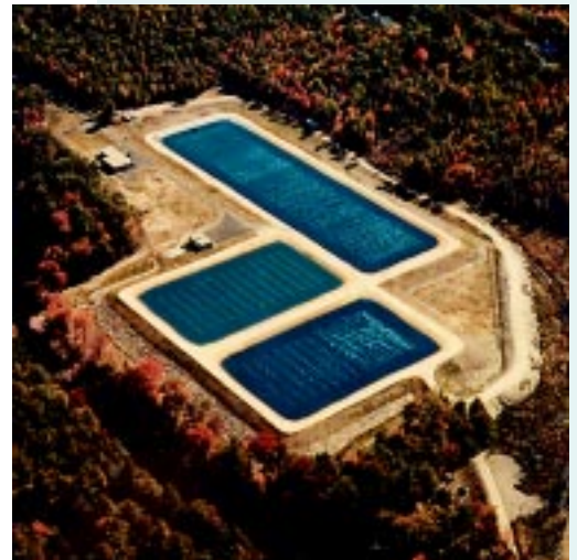
Facultative sewage lagoons utilizing the Ozonex aeration system require less detention time and use less energy.
