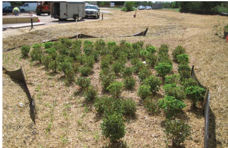
Above: Planted Infiltration Basin
