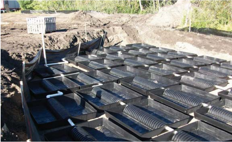
Below: Sand Base Rootzone Installation
