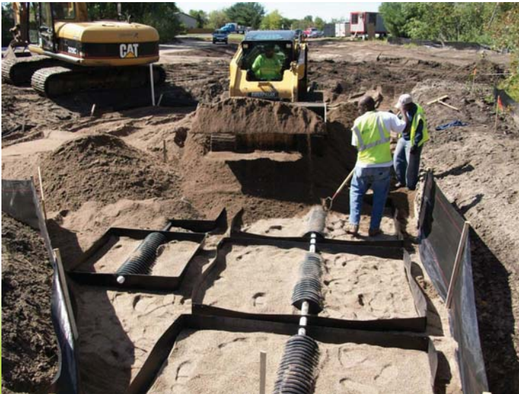
Below: Sand Base Rootzone Installation
